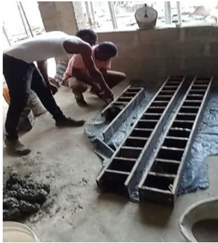
Plate 4: Concrete Cubes Formwork
