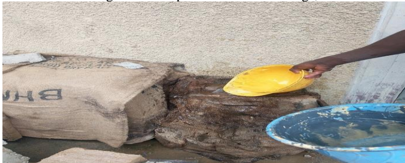
Plate 4 Curing of Slab with Wet Jute Bags
