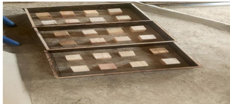
Plate 1 Formwork for waffle slab with wood edges and wooden pods
