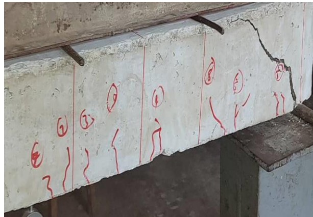
Plate 6: Cracks on beam during flexural test
