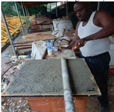
Figure 2.5 Casting and vibration process
