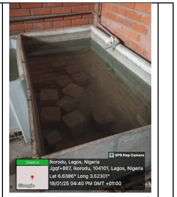
Figure 16: Curing of concrete
